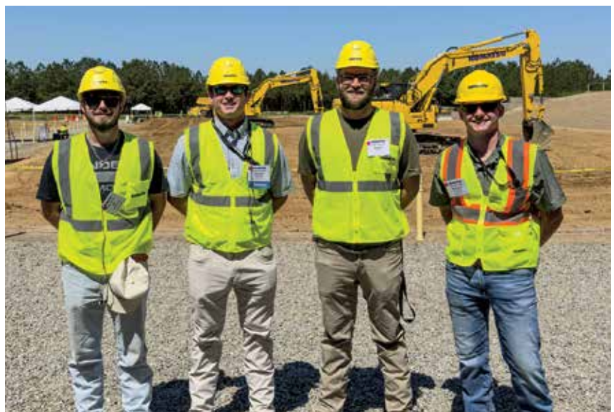
(L-R) Pruitt Excavation's Ian Underwood, TEC's Conner Bussman, Pruitt Excavation's Austin Pruitt and Rox Plus's Bransen Anderton check out Komatsu excavators.
