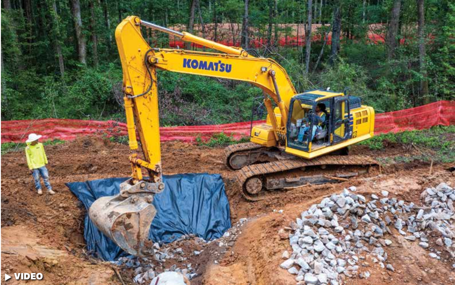
An operator lays stone for a utility installation using a Komatsu PC290LCi-11 IMC excavator.
