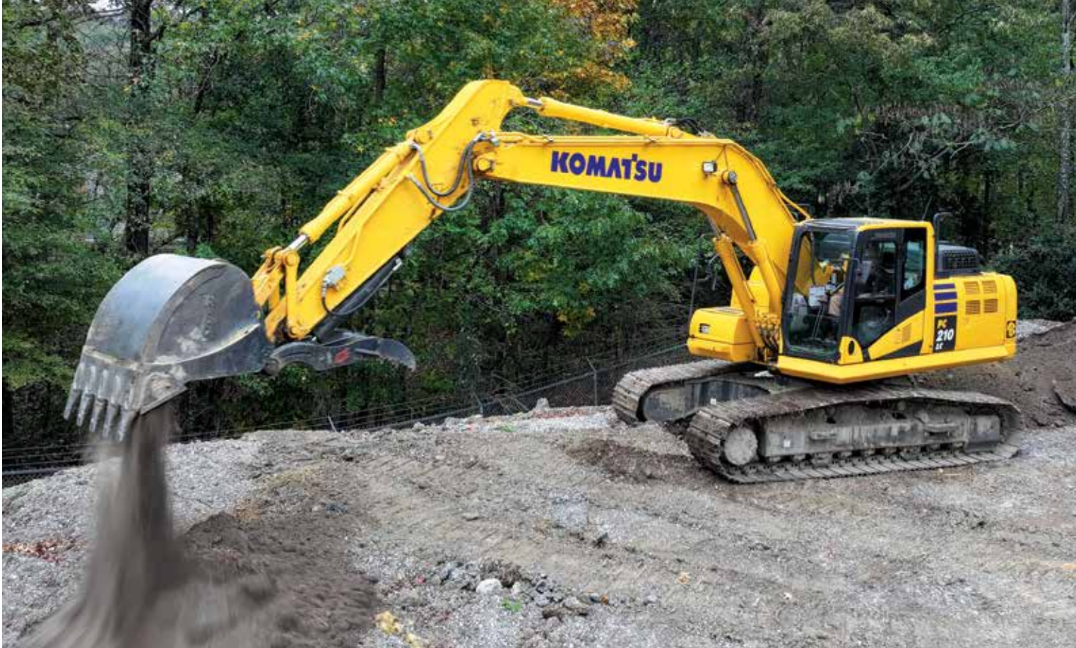
Project Manager Noah Egan moves material at the North Shelby Wastewater Treatment Plant with a Komatsu PC210LC-11 excavator.
