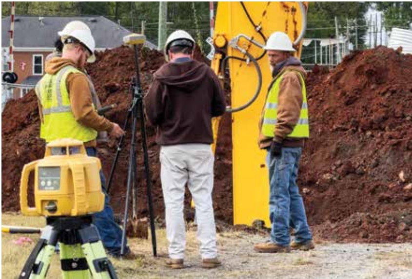
David Gilleland (center) verifies grade depth and width using a base and rover station.
