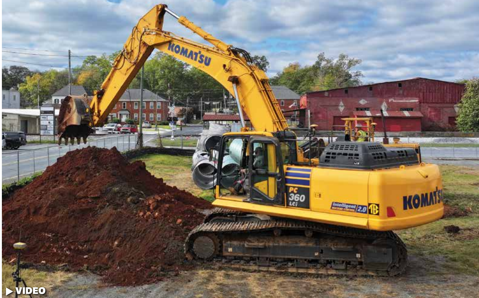
An operator uses a Komatsu PC360LCi-11 intelligent machine control (IMC) excavator to cut a ditch to grade for a new pipe installation at a project in Cartersville, Ga.
