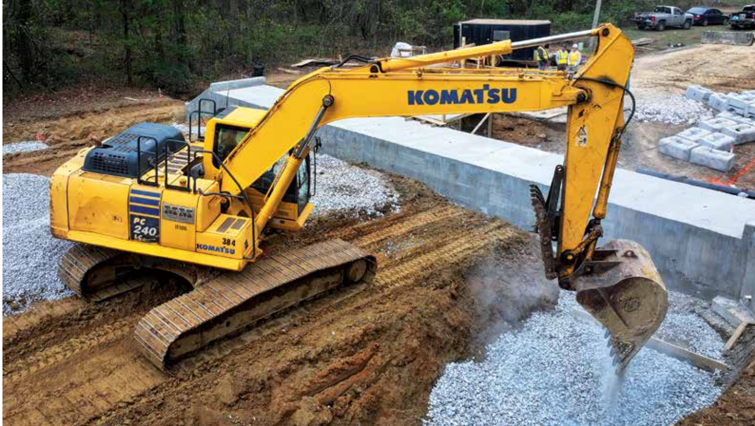
An operator places base rock with a Komatsu PC240LC excavator at a box culvert job.
