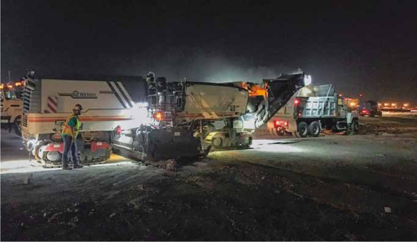
An Atlanta Paving & Concrete Construction crew works at night to complete a milling project at the Hartsfield-Jackson Atlanta International Airport.
