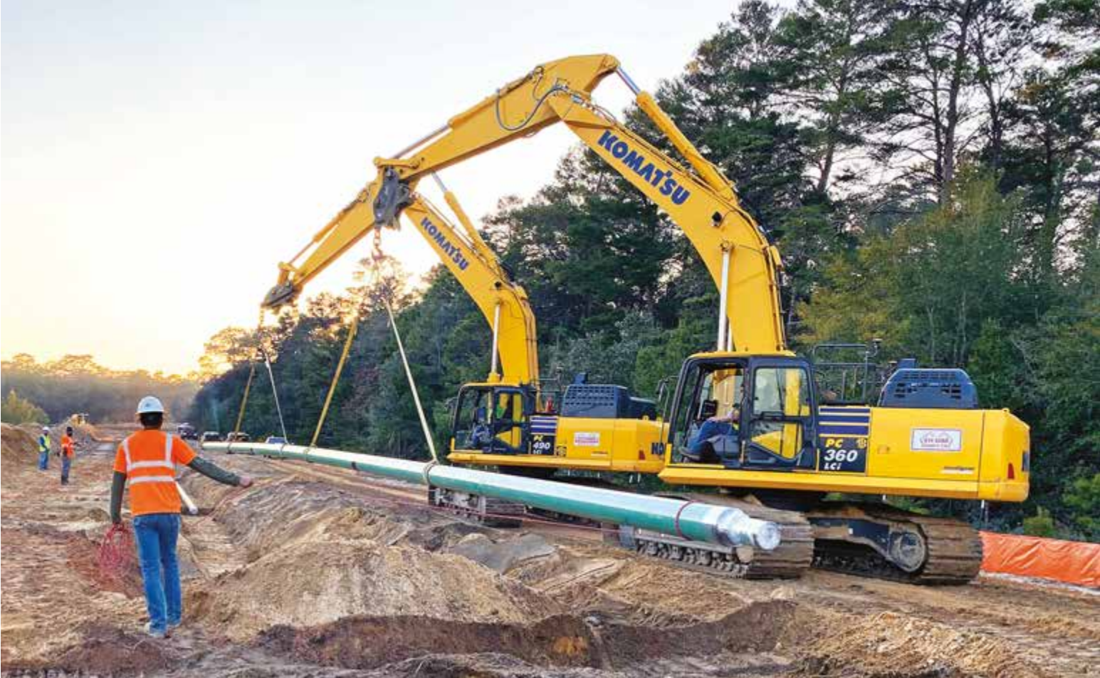
814 Sand operators place pipe in a trench using a Komatsu PC360LCi-11 excavator and PC490LCi-11 excavator at Eglin Air Force Base in the Florida Panhandle. “Everything on the project is also sloped on a precise uphill and downhill grade to create gravity flow,” said Superintendent/Project Manager Stan Pitts. “The intelligent GPS equipment comes in handy for putting everything on grade; we know we’ll be on the money.”
